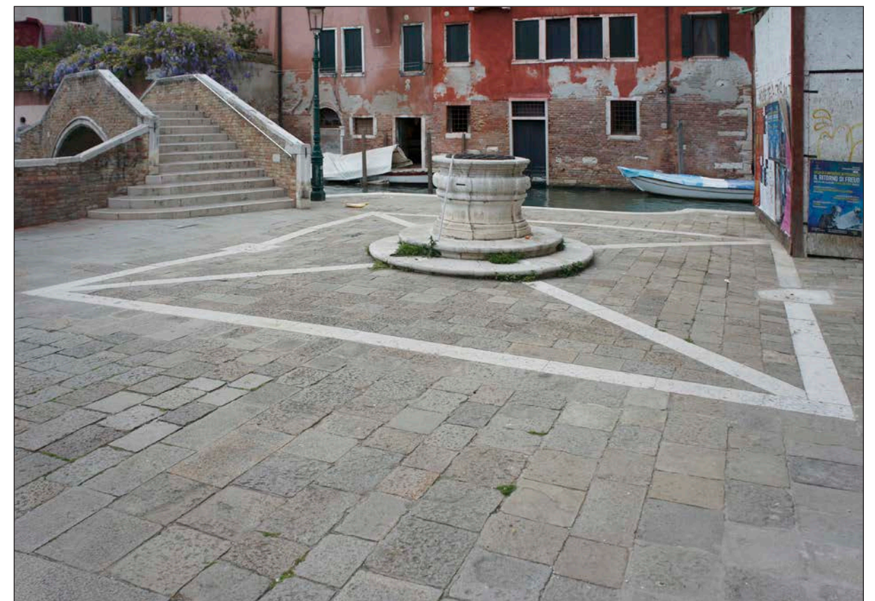
Fig 32. Oligocene trachyte/Jurassic Istrian limestone field with Istrian well head over Holocene sand hydrologic basin.
