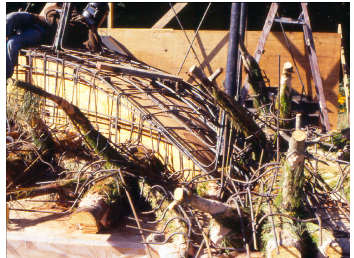
Fig. 176. Humboldt Ship, construction of core element on horizontal platform, 15 ft. x 22 ft.. wood, sawn pine logs, clay, pine needles, steel support tubes, rebar.
