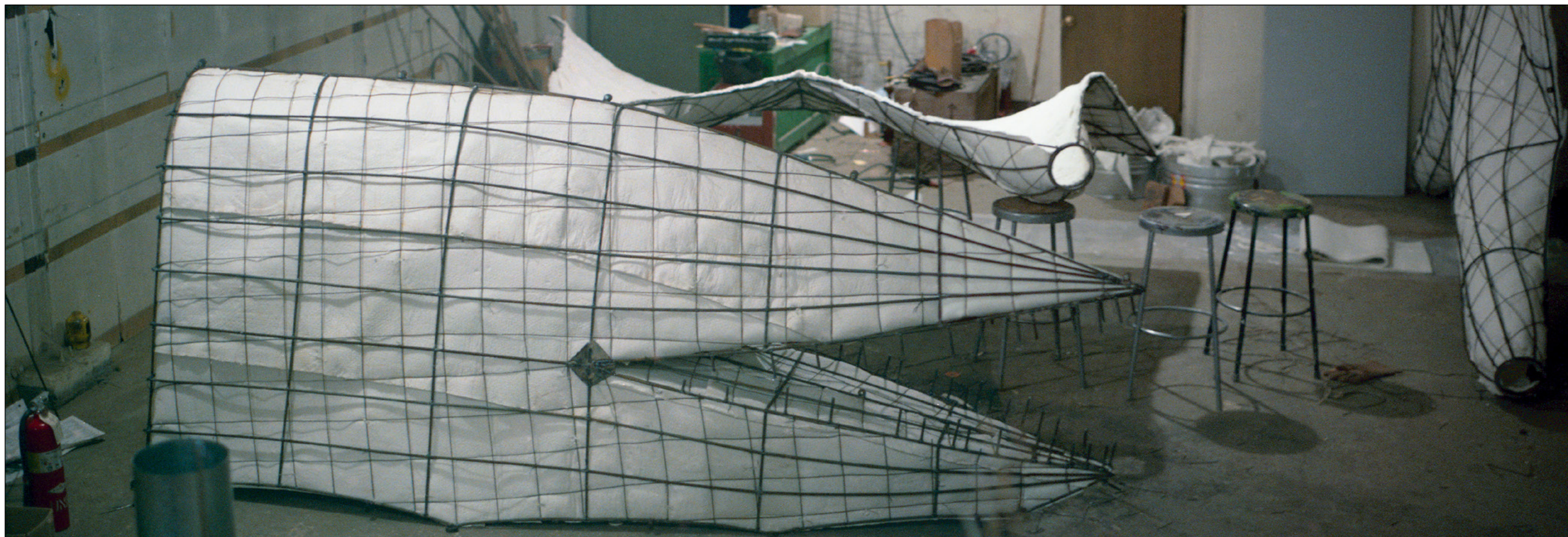
Fig 131. Fabrication of kiln components, steel, ceramic fiber blanket, sculpture shop, University of Nevada, Reno. Flue/fish eye ports for exhaust stacks added after this image was taken.
