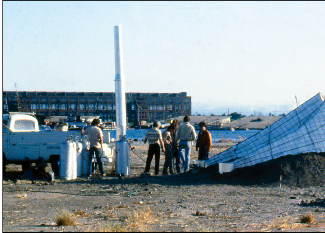
Fig. 316. Mountain Kiln/Black Orchid . Crew members hooking up the propane tanks and installing the burner system.
