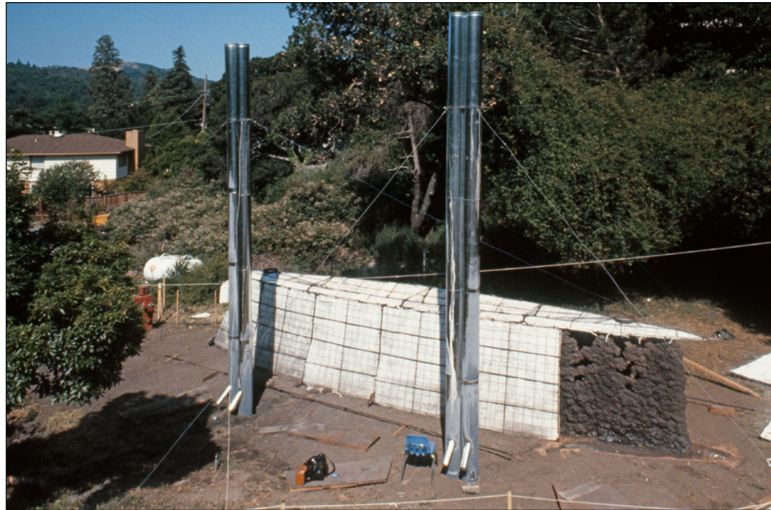
Fig. 105. Collision: Lava Ship / Trellis Ship (post firing/Fused State), dismantling of kiln.
