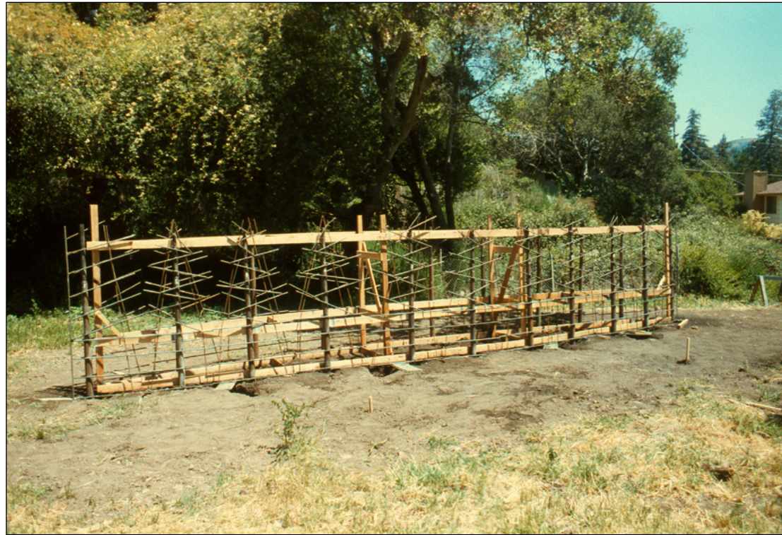
Fig. 98. Site installation of Lava Ship's internal steel pipe armature.
