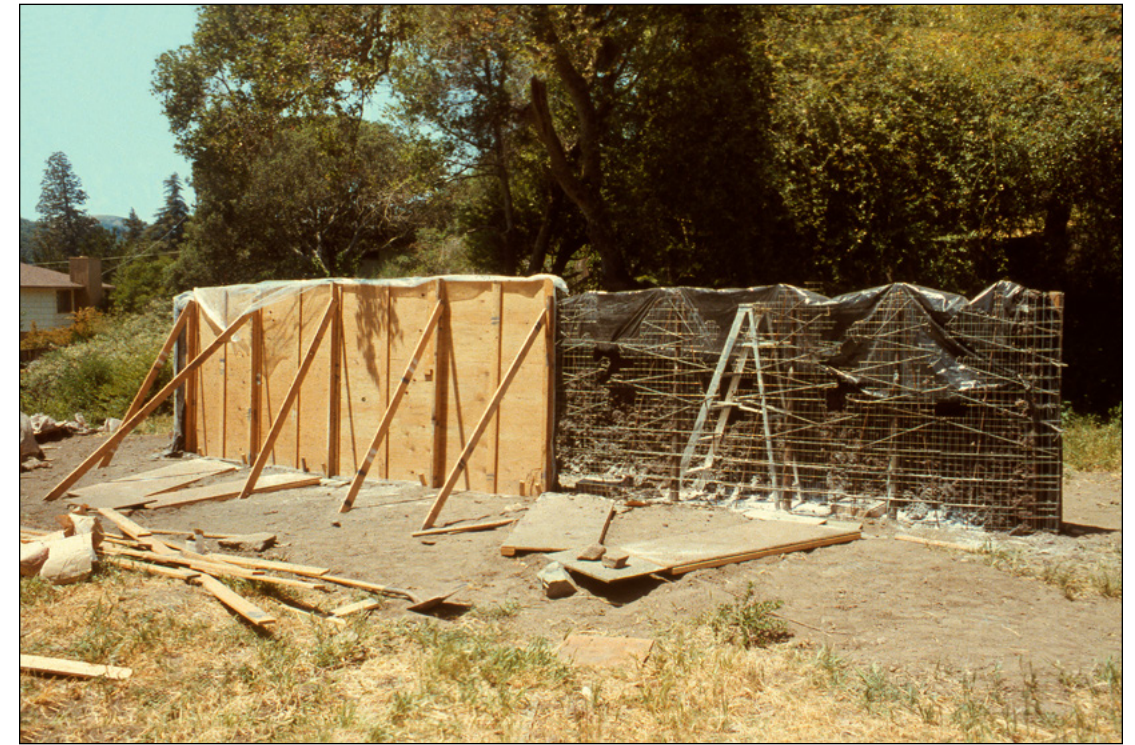
Fig. 100. Lava Ship , construction of mold element for placement of clay around the ship's steel armature.
