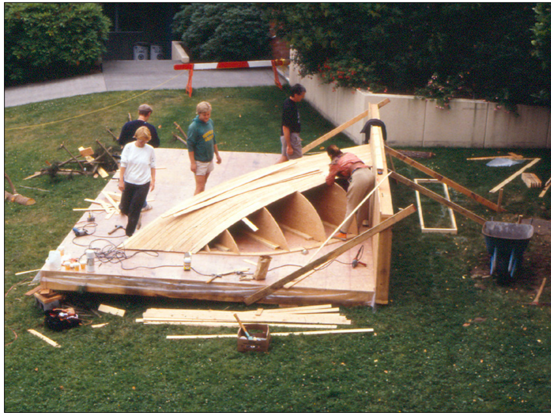
Fig. 174. Humboldt Ship, construction of core element on horizontal platform, 15 ft. x 22 ft.. wood.
