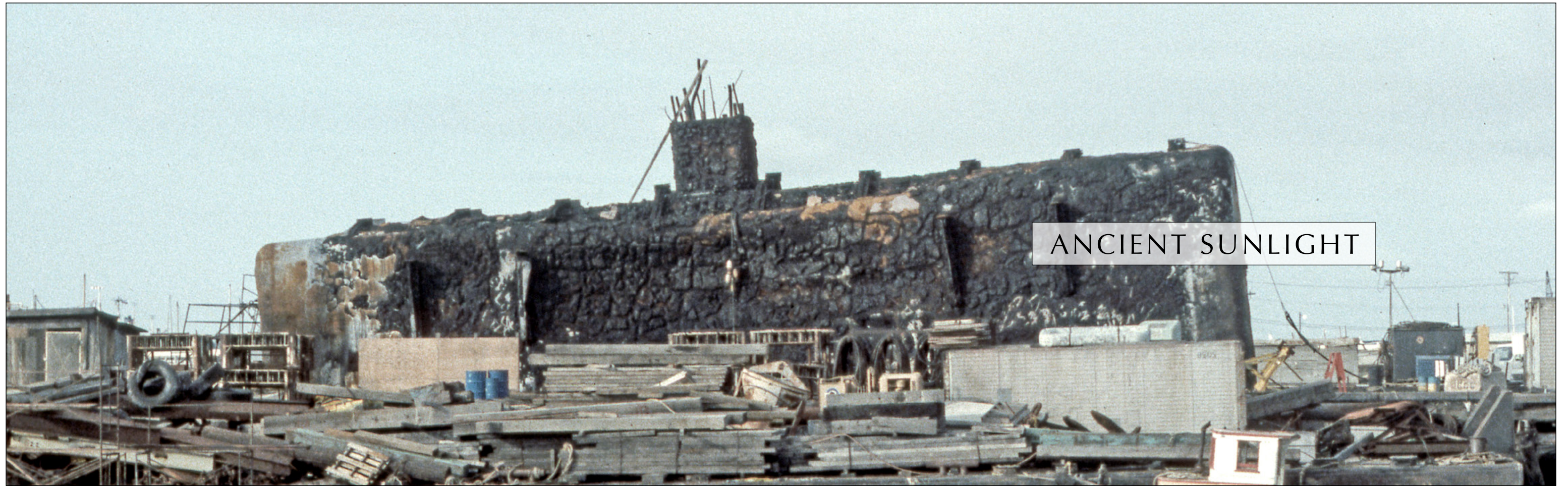
Fig. 274. Derelict fuel bunker, estuary, Oakland, CA, circa 1985.
