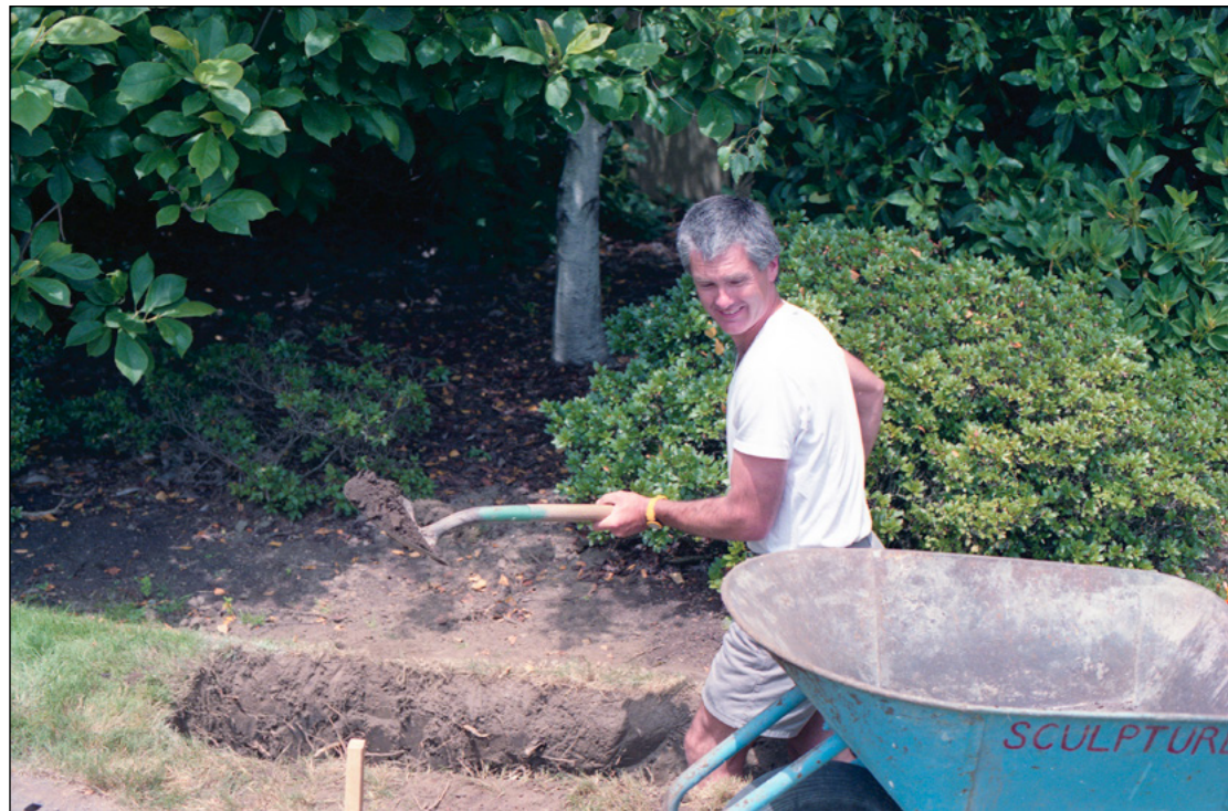
Fig. 326. Humboldt Ship , . Jim Crawford, Art Department Faculty, at work digging trench for cement kiln foundation.
